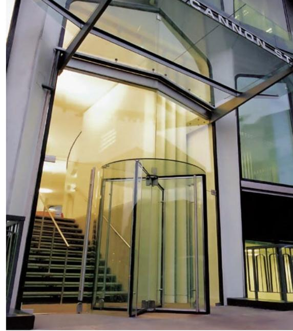
The Crystal TQ uses a combination of tempered and laminated safety glass. The doorset is made from 1/2" tempered glass connected to the center stainless steel shaft with specially made stainless steel clamps. The 11/16" tempered laminated glass ceiling is fixed directly to the curved laminated glass sidewalls with small, unobtrusive clamps. Tinted glass is available.
